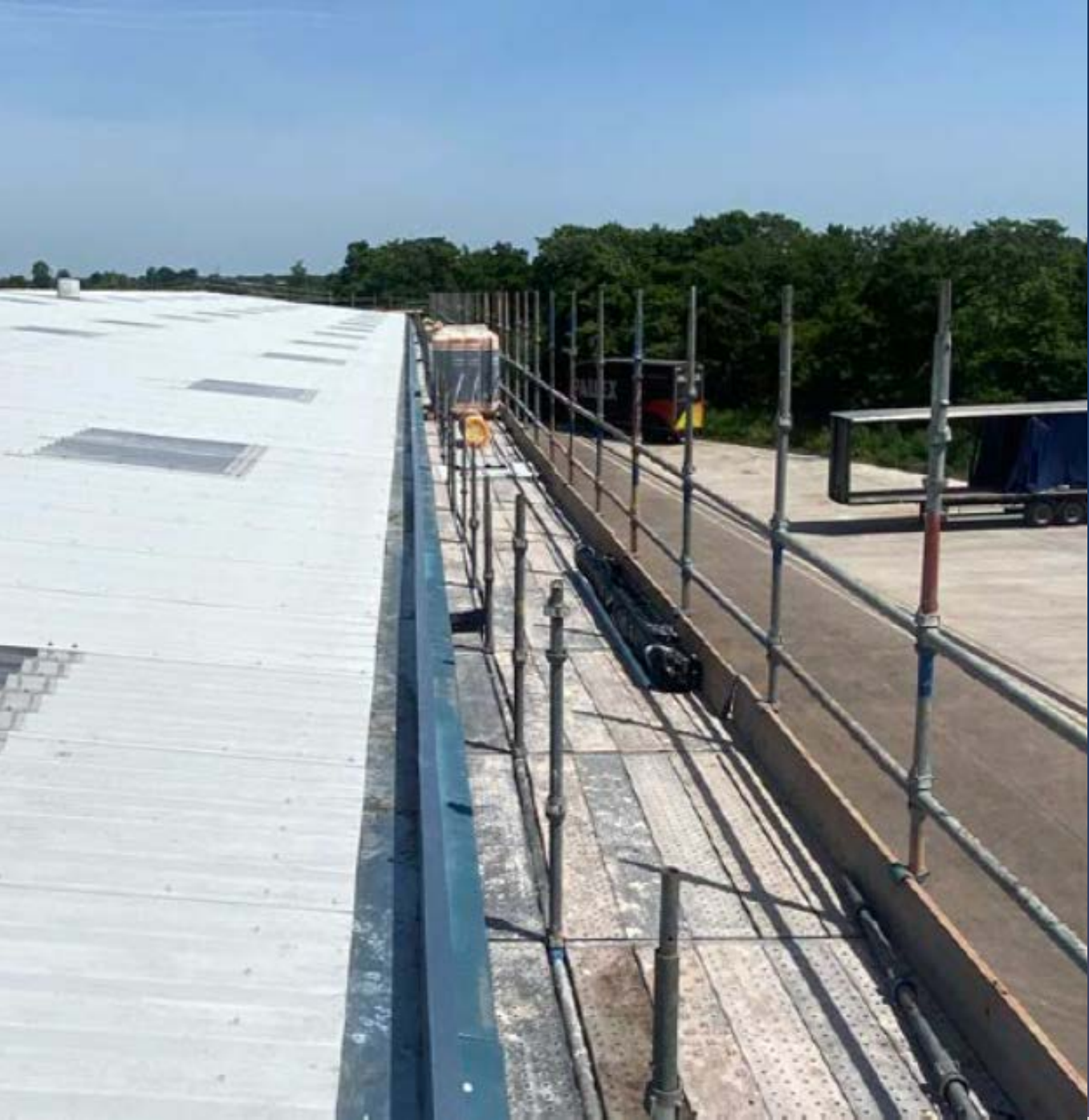
Fortec Distribution Centre WIP
