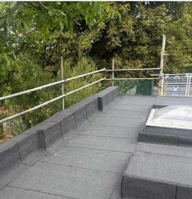
Groveside School, Reading (Felt Upstand Detailing)
